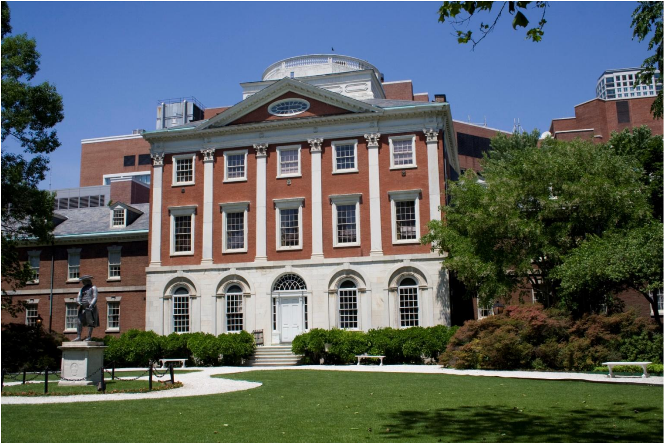
Pennsylvania Hospital in Philadelphia, PA, is the nation's first hospital and on the National Register of Historic Places
